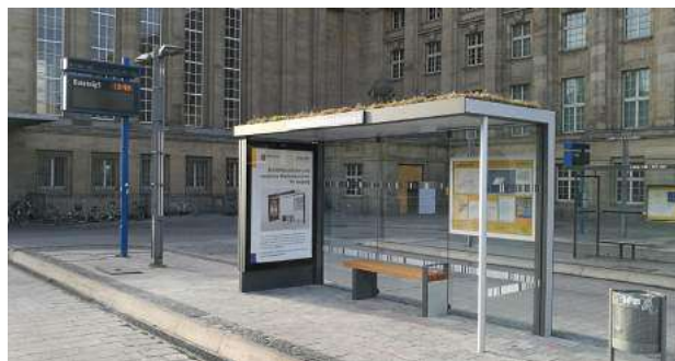
Wartehalle Progress in Leipzig
